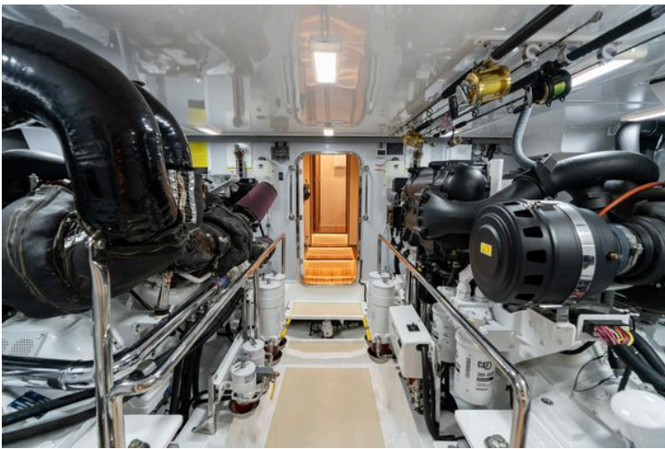
Engine Room Facing Fwd
