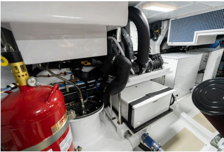
Engine Room Facing Stbd
