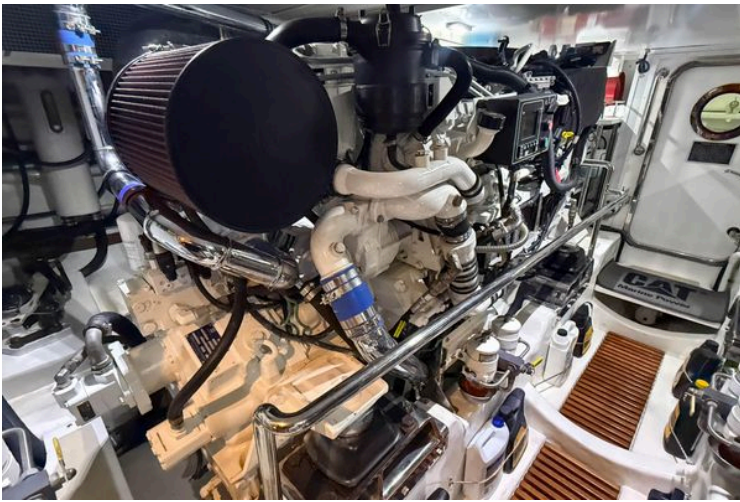
Engine room of 2018 Marlow 53E yacht, featuring advanced marine power systems.
