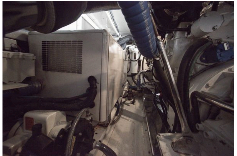
Engine room of 2009 Marlow 78E yacht with complex machinery and cables.
