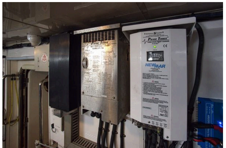
Electrical equipment in a 2009 Marlow 78E yacht engine room, featuring a Newmar smart charger.
