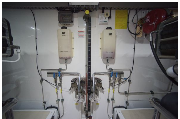
Forward Engine Room Wall, Fuel Manifold
