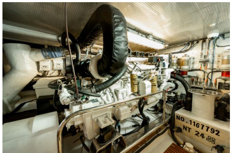
Engine Room Port
