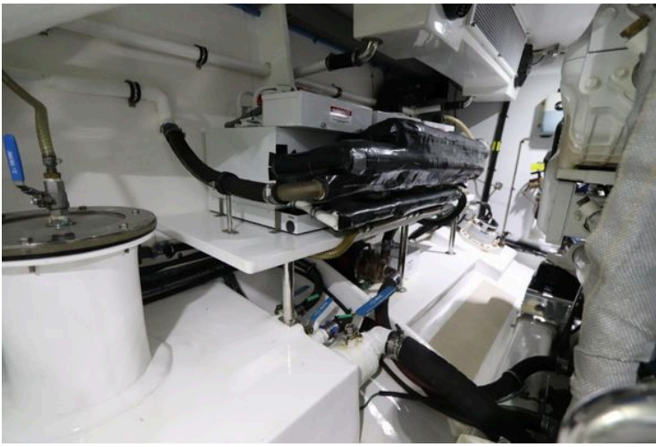
Engine room of 2017 Marlow Explorer 49E yacht, showcasing mechanical components and piping.
