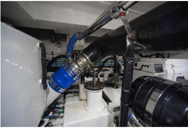
Engine room of 2013 Marlow Explorer 62E yacht, featuring pipes and machinery.
