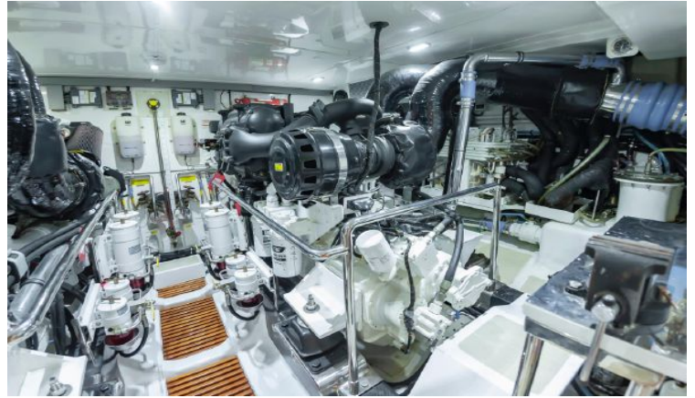
Engine Room facing Starboard
